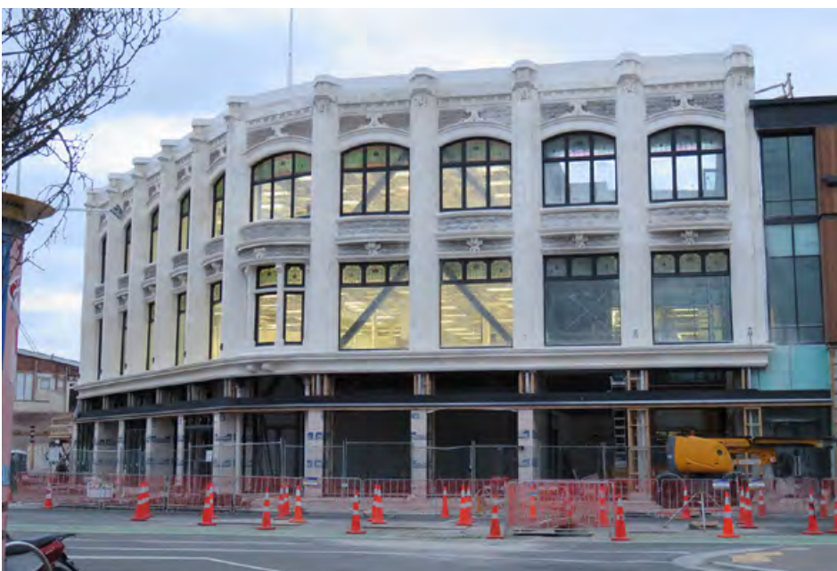
Fig. 15. Restored façade with construction of new building occurring behind. The steel braces supporting are clearly visible through the windows (Source: C. Forbes, 13 September 2016)
