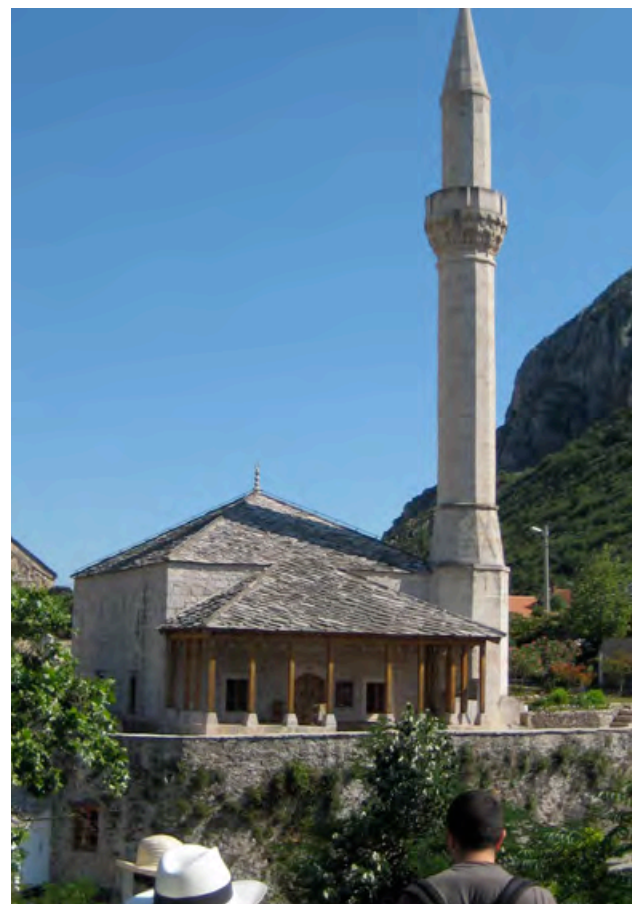
Fig. 10. Nezir Aga Mosque from the north, after reconstruction
