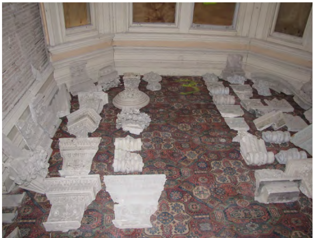
► Fig. 30. Plaster brackets have been salvaged, sorted, inventoried and stored for future reinstatement (Source: CCC 25/3/2019)
