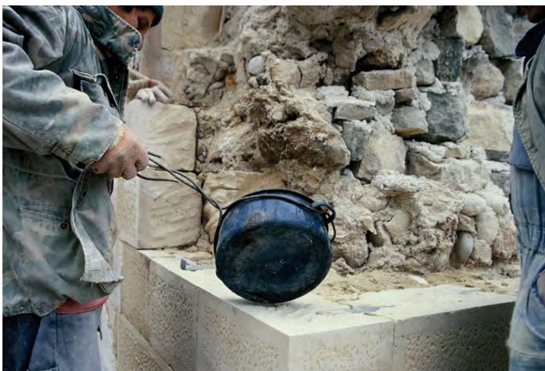
▲ From top to bottom: Fig. 27. Starting to work on the qibla wall Fig. 28. Pouring molten lead to fix a clamp
