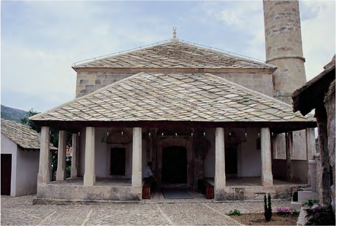
Fig. 29. View from the north after restoration
