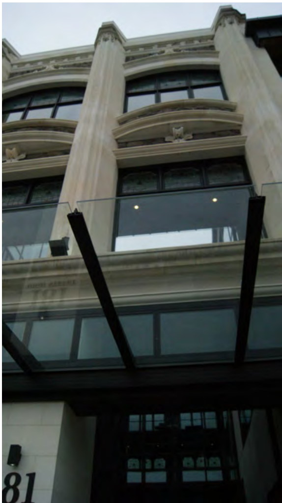
Fig. 19. The new glass awning over the footpath and new shop fronts (Source: A. Ohs, 21 November 2019)
