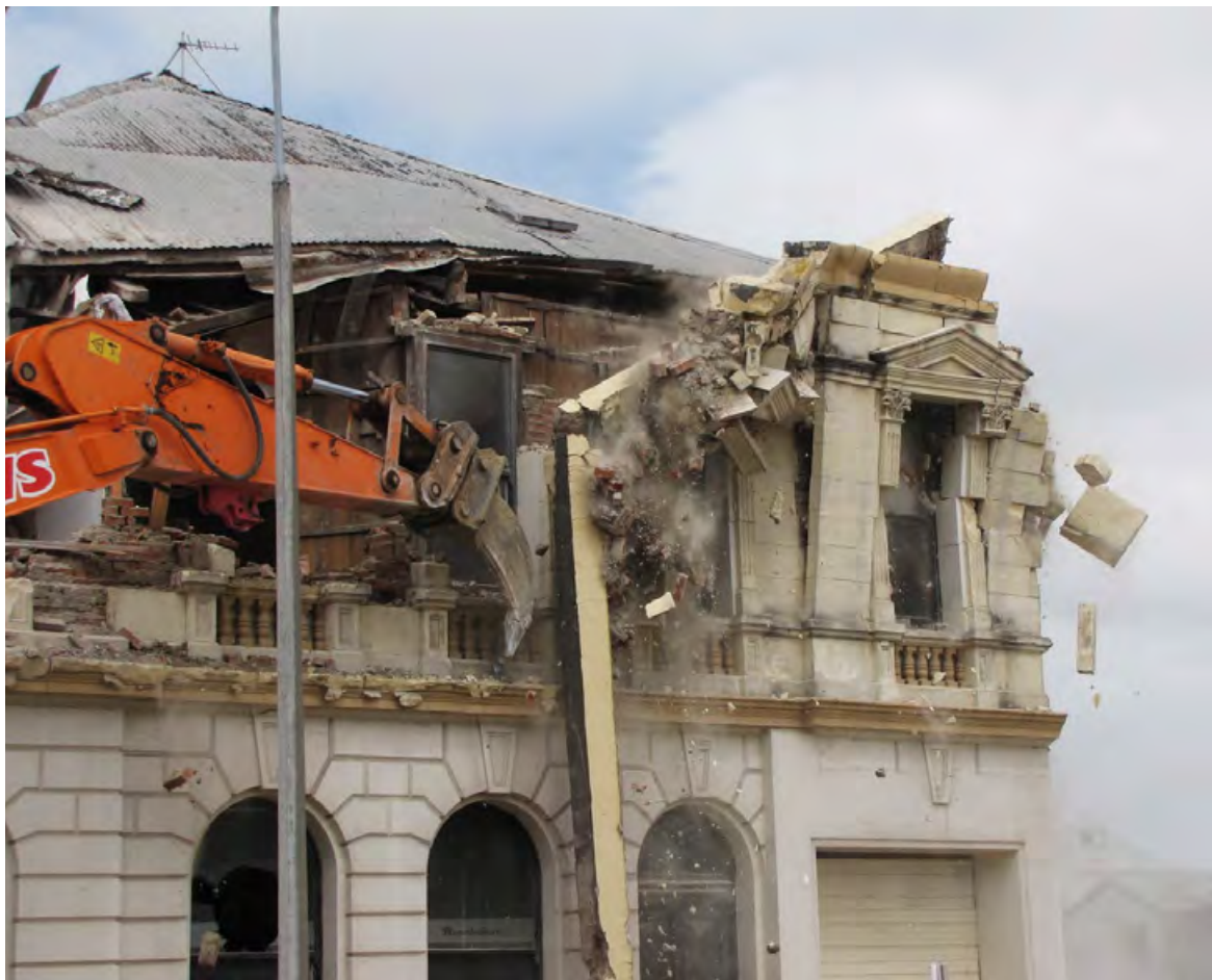
Fig. 24. Demolition in progress of 136 Lichfield Street, central Christchurch (Source: B. Smyth, 29 February 2012)
