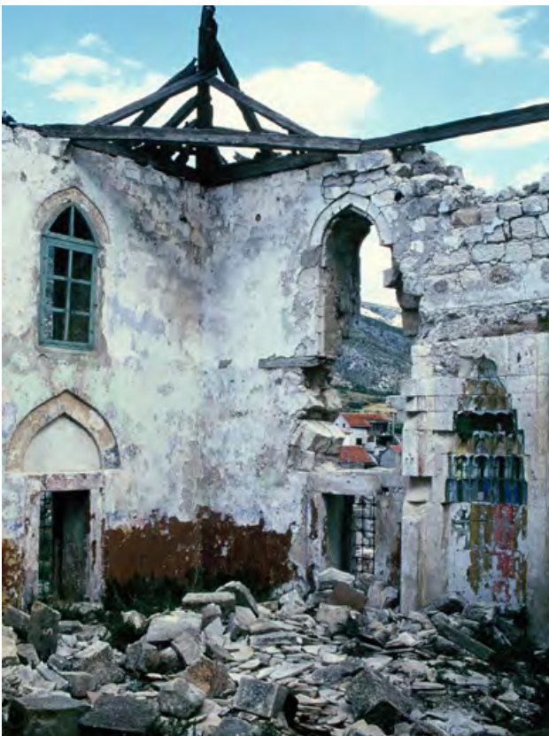
Fig. 14. Sevri Hadzi Hasan Mosque, the northeast corner of the roof
