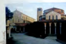
Facade of Santa Fosca, Torcello
