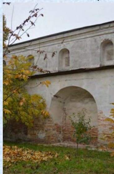
Fixation of destruction of the front surface of the walls at the site No1 Monastery Walls
