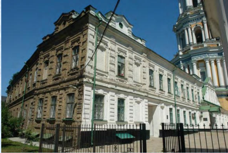
Southeast corner of the building
