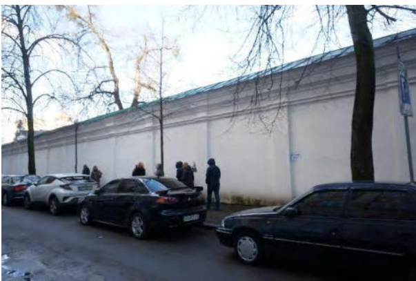
The renovated part of the surrounding wall -
