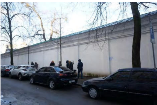
The renovated part of the surrounding wall -
