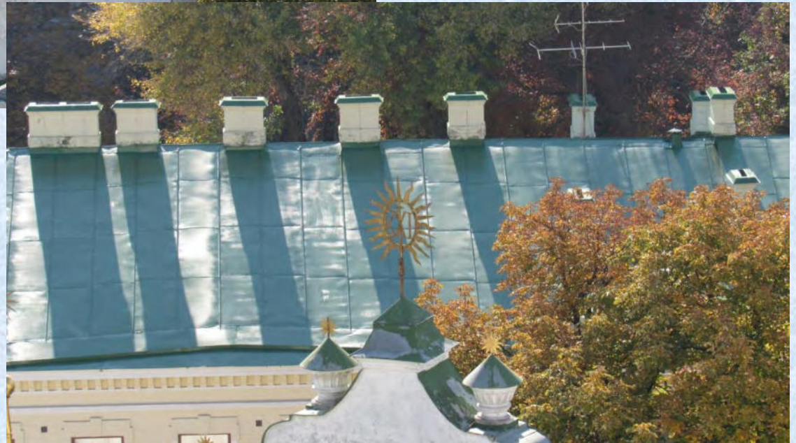
Ongoing repair of the roof
