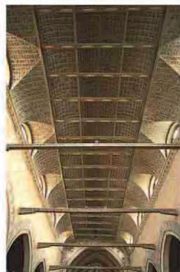
The ceiling of Santo Stefano, in the form of a ship's keel
