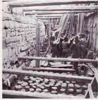
Strengthening the Campanile foundations
