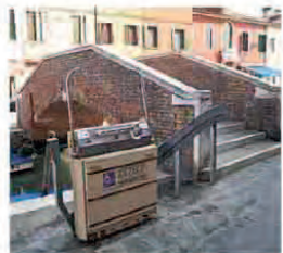
A mechanically operated wheelchair ramp across a bridge
